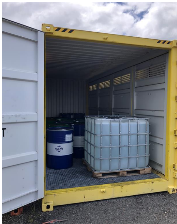
Figure 12 – Bunded chemical storage container
