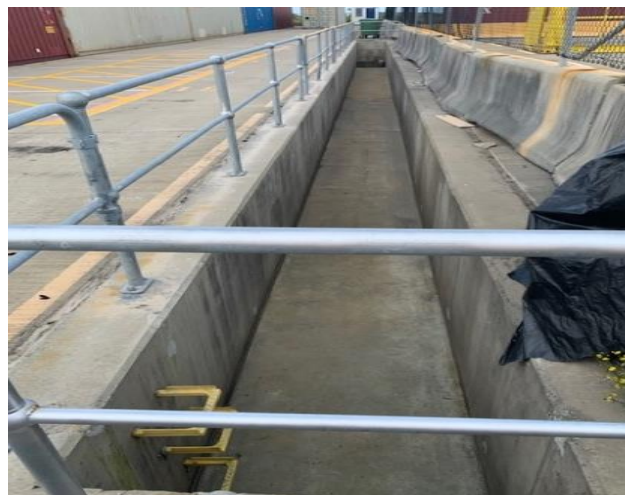
Figure 11 – Stormwater drain at the R area cleaned out
