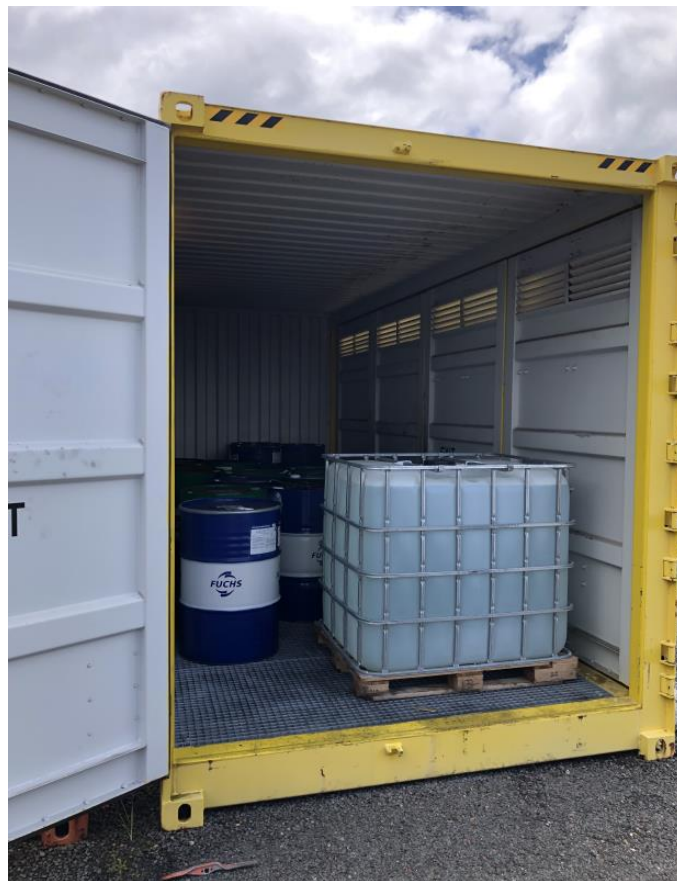
Figure 12 – Bunded chemical storage container
