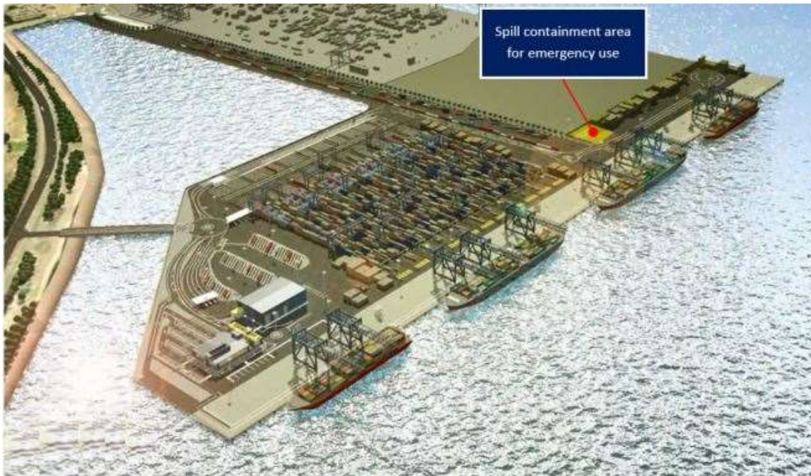
Figure 15 Location of Spill containment area
