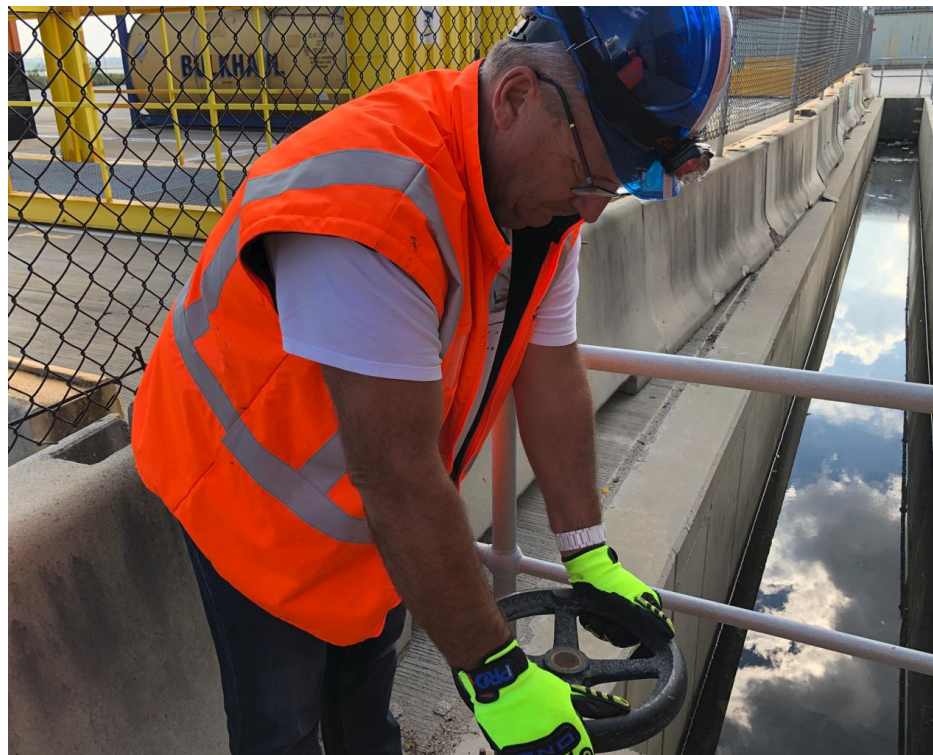
Figure 11 - Closing of the emergency shut-off valve during the drill
