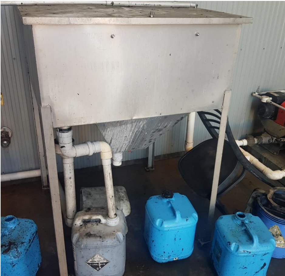
Photo 5: Waste oil separator
