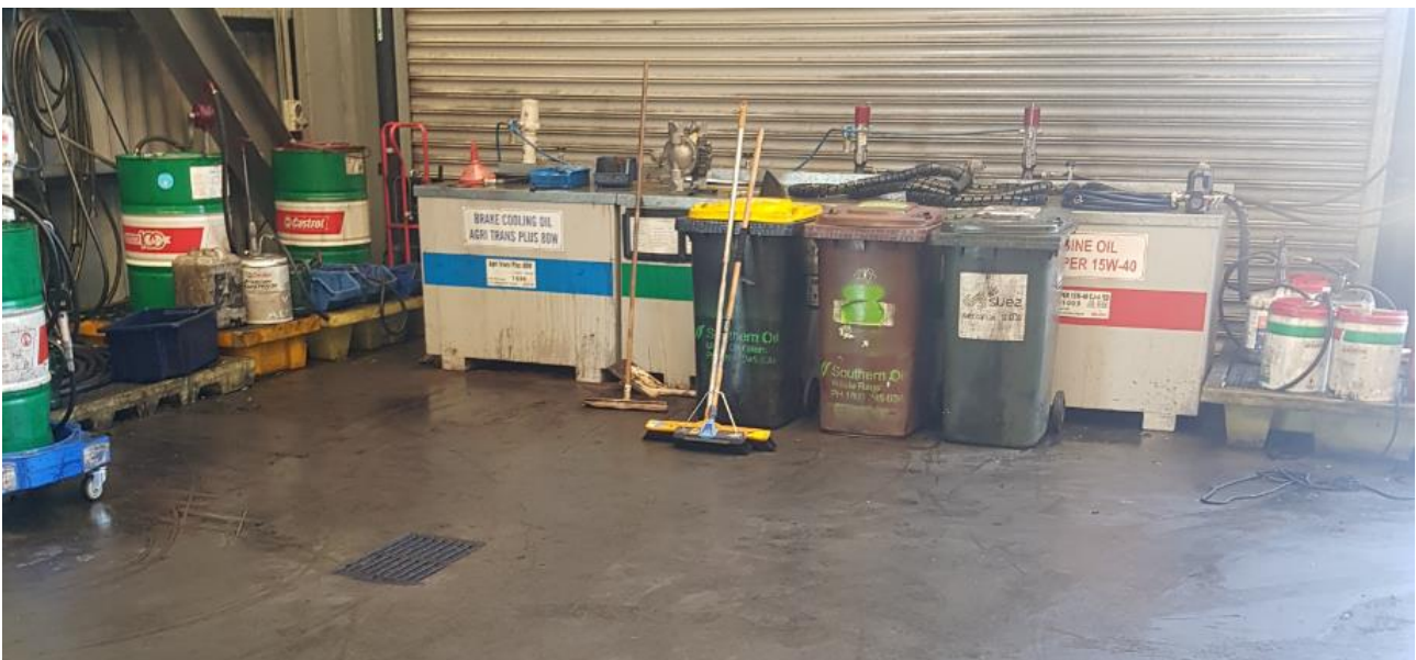
Photo 6: Liquid storage within the sealed and banded maintenance building. The drain in shot does not flow to environment.
