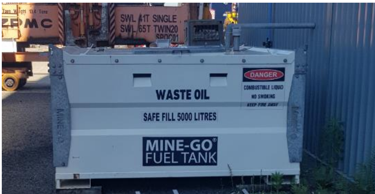
Photo 9: The self-bunded waste oil unit.
