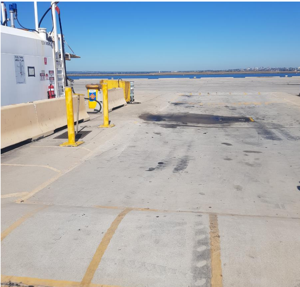
Photo 11: The contained refuelling bay (with 67kL tank to left of shot, bund, blind central pit and spill kit).
