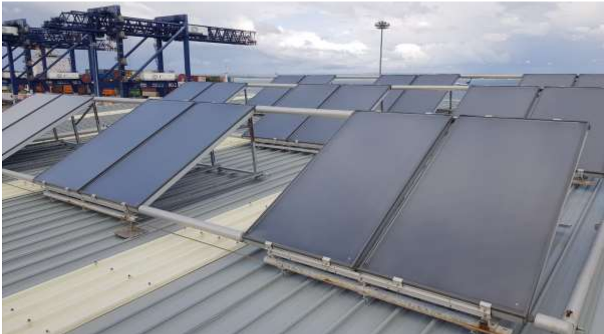
Photo 5: Solar panels servicing the maintenance building
