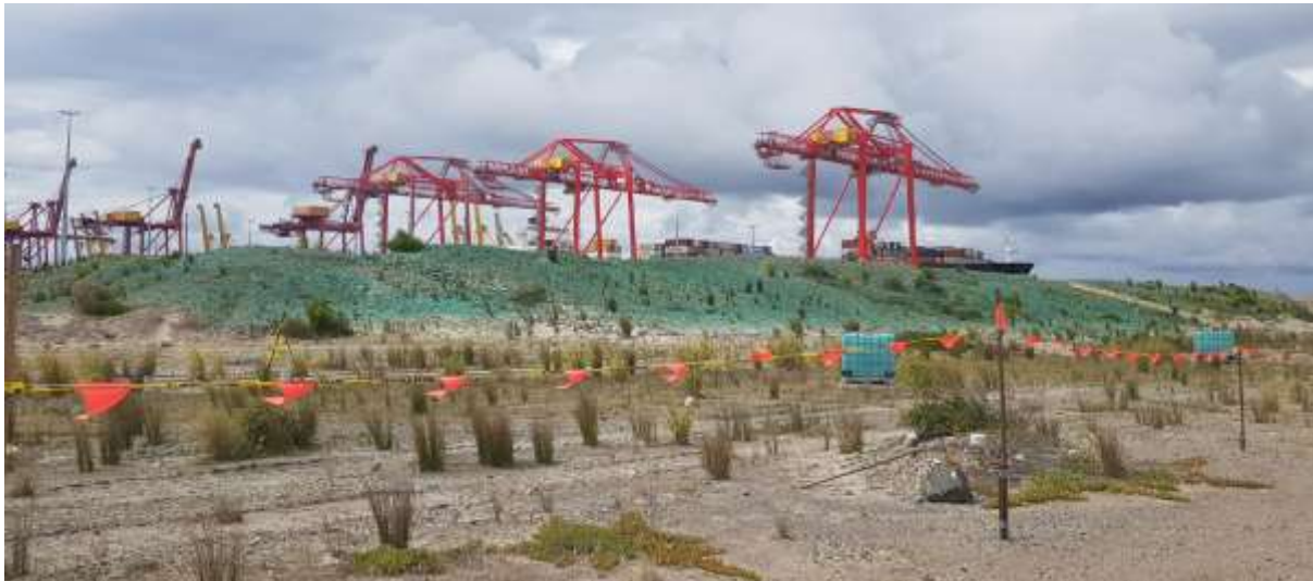
Photo 11: Stabilised stockpile in Phase 3 area.
