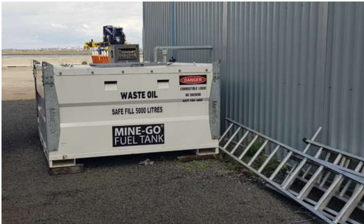
Photo 9: Maintenance shed waste oil unit.
