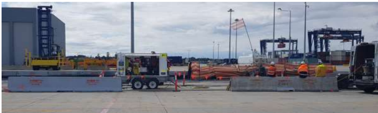
Photo 10: Stormwater clean out works in progress.
