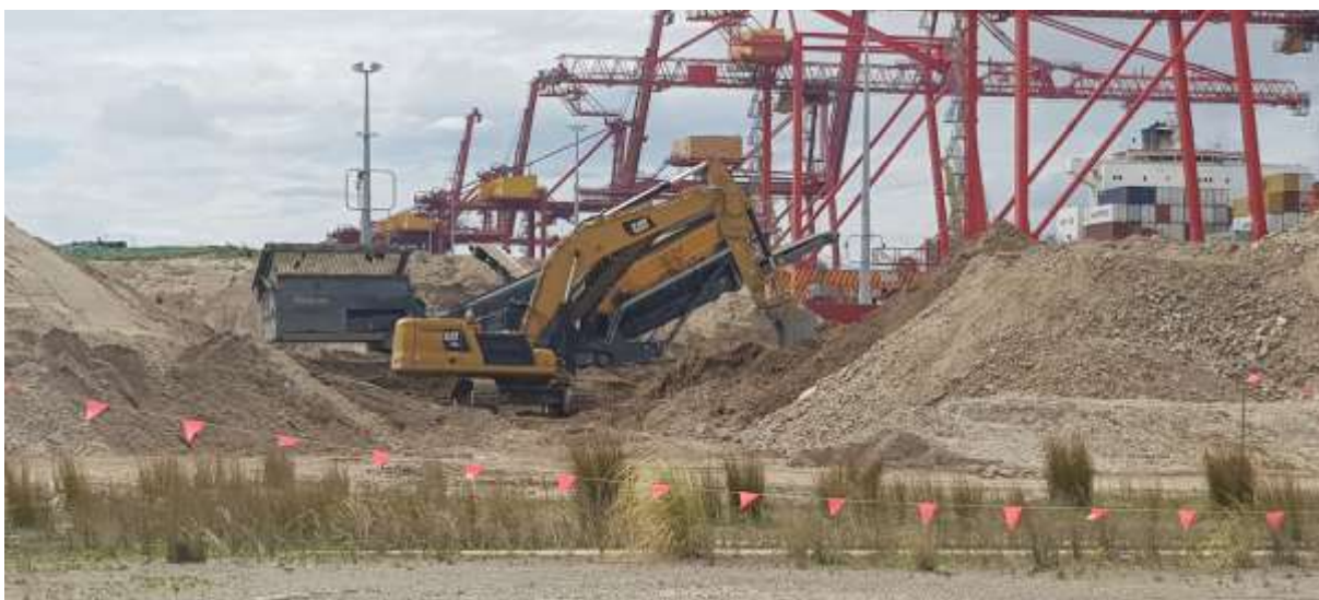
Photo 12: Stockpile removal works in progress (no issues).
