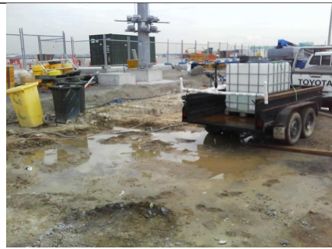
Photo GC6 Water cart used for dust suppression
