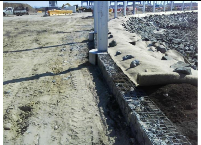
Photo LO20 – Foundations and early phase of installation of noise wall
