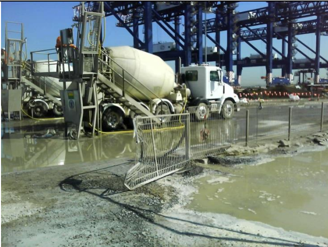
Photo LOR13 – Boral batch plant – concrete washout area. Concrete washout generally well managed across the site.
