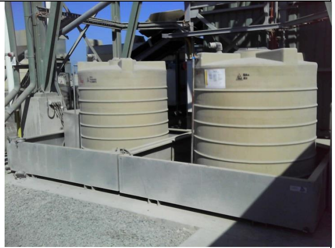
Photo LOR14 – Appropriate bunded storage of concrete additives at the Boral Batch Plant
