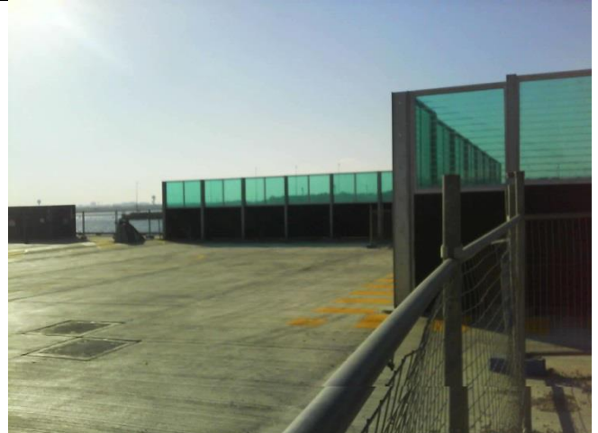
Photo LOR21 – Completed section of noise wall
