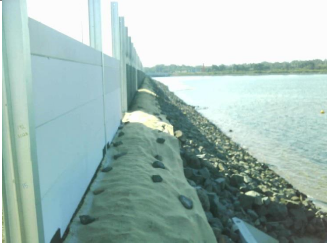
Photo LOR21 Installation of noise wall
