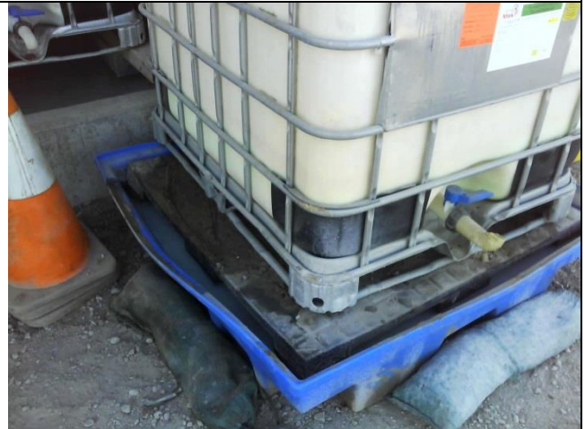
Photo LOR 2: Bunded pallet full of water (no capacity for spillage)
