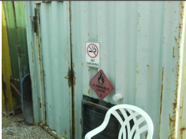
Photo GC1: Hazardous storage container – in poor condition with rust holes and no built in secondary containment
