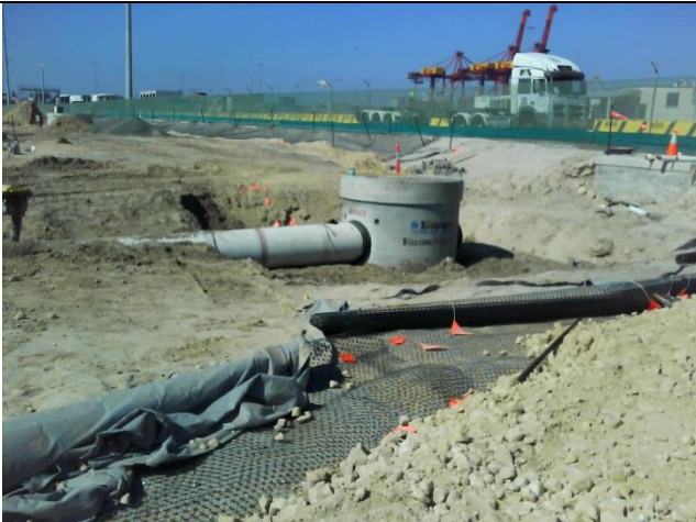
Photo LOR7: Installation of Stormwater devices
