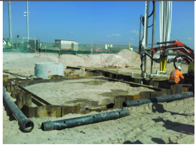
Photo LOR8: Installation of SQID. Groundwater is pumped out into tanks and discharged to the bay only after water quality is checked.
