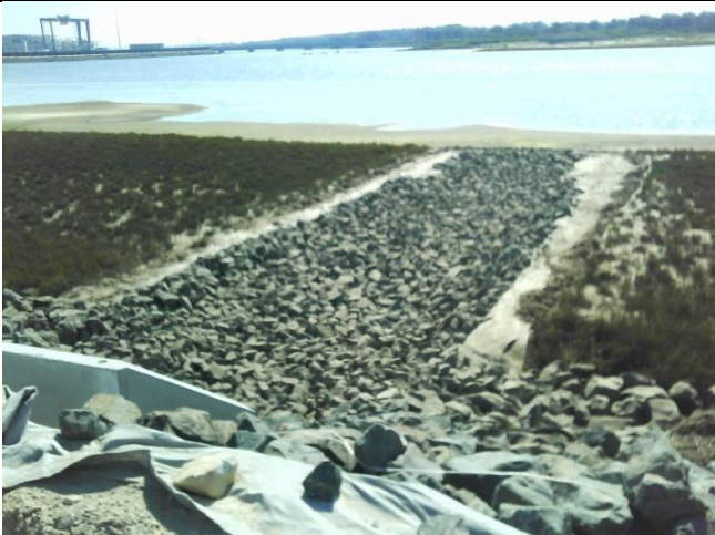
Photo LOR9 – Rock lined channel under construction – discharge of stormwater. Saltmarsh removed was planted elsewhere.
