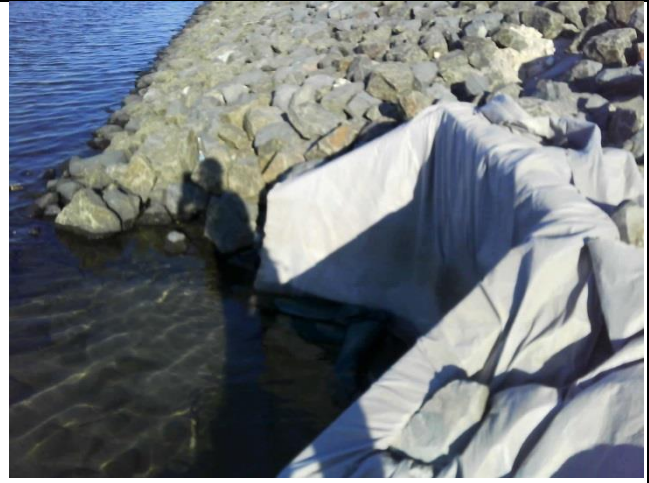
Photo LOR10 – Protected drain (thick geofabric) – interim measure until SQIDs fully operational
