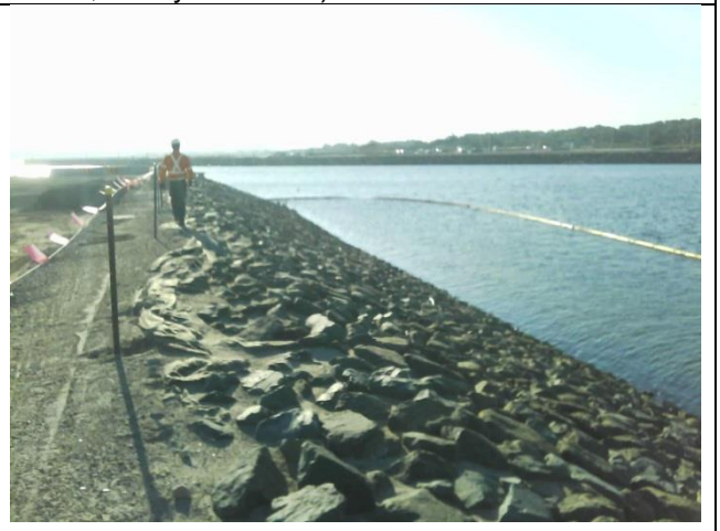
Photo LOR6: Short section of silt curtain underwater (top RHS of curtain). Needed repair
