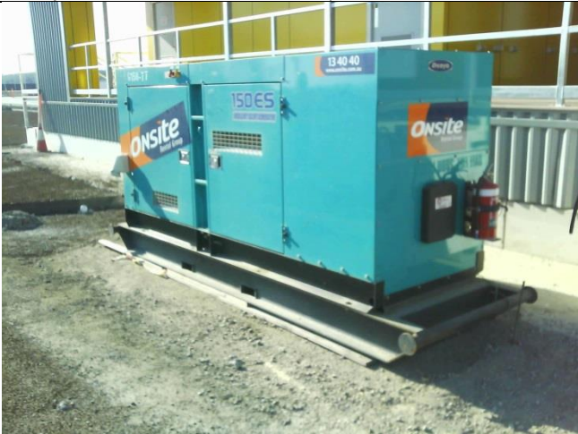
Photo LOR19 – Fuels on site are stored within double skinned storage tanks. Bowser kept locked. (this container about to be moved)
