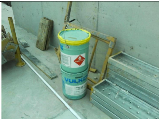
Photo GC5: Containers of chemicals ready for use stored in building under construction. Appropriate MSDSs not available and personnel unsure of disposal requirements for container (DGs)
