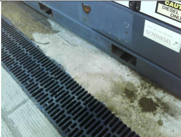
Photo KC3 – Evidence of minor leaks of diesel into stormwater drains.
