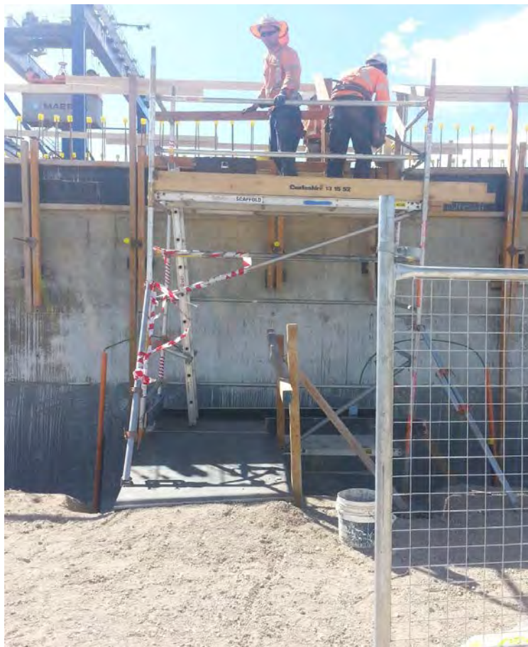
Photo 003: Substation scaffolding with no scaff tag and not tied in to the wall.
