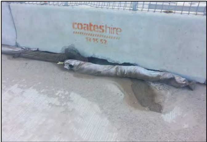
Photo 002: Example of silt sock in need of attention and build up of sediment.
