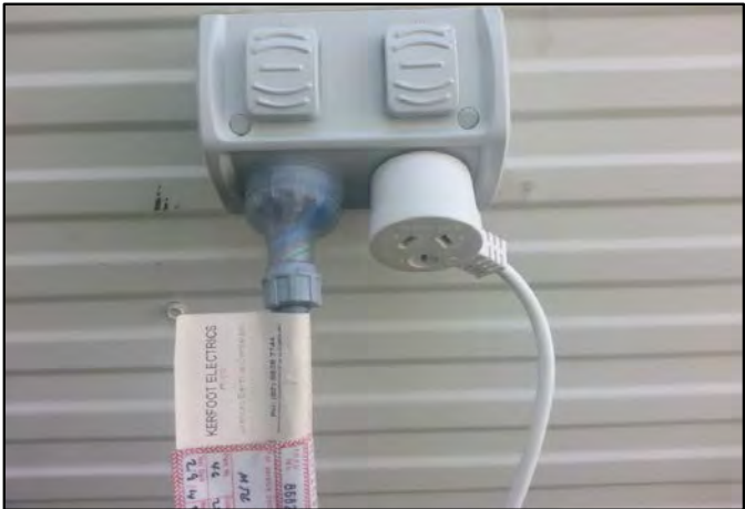
Photo 001: IP53 plug (right) used to power vending machine plugged into an outside outlet which is exposed to rain.
