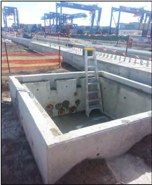
Photo 004: Example of one of the unsafe ladders in use. This example shows the primary access and egress ladder to this pit is not anchored in anyway.
