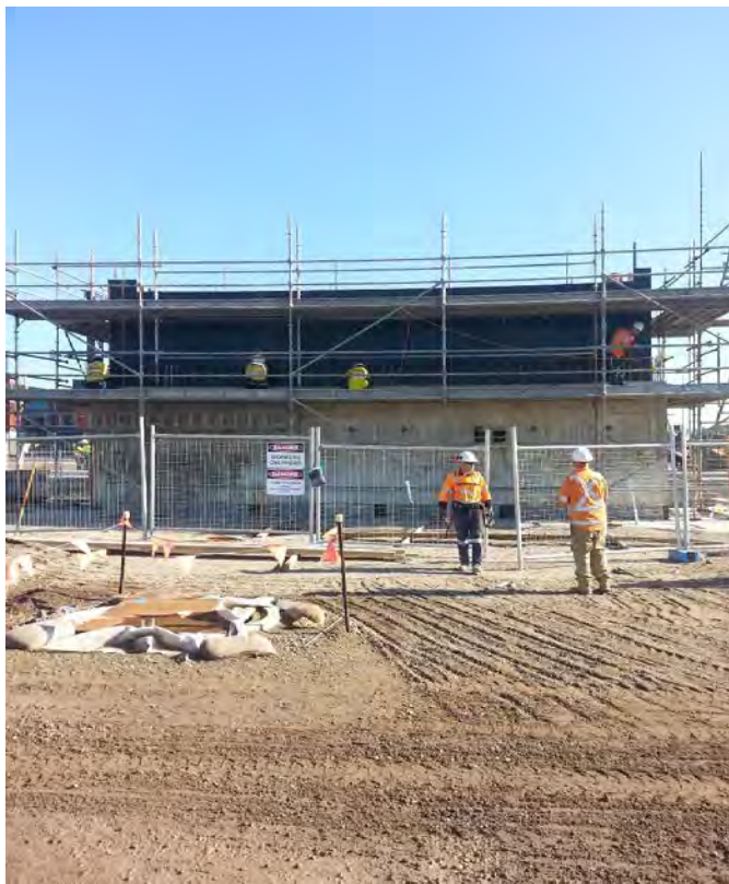
Photo001: The new standard of scaffold used at Port Botany. KNF have subcontracted the work to a professional installation company and the quality has improved 10 fold. Note the kickboards, longitudinal bracing, access stairs, mid and guard rails. Well-done.
