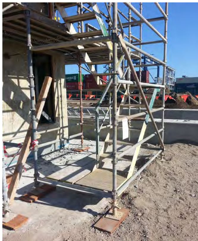
Photo002: Safe access and egress from the scaffold now possible. Scaffold tag in place, but not ideal. Perhaps an opportunity for improvement on behalf of the subcontractor ACROW (tag appears to be missing the next 30 day inspection date).
