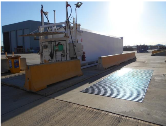
Spill Kit and the tray and grate bunding system at the diesel fuelling station.
