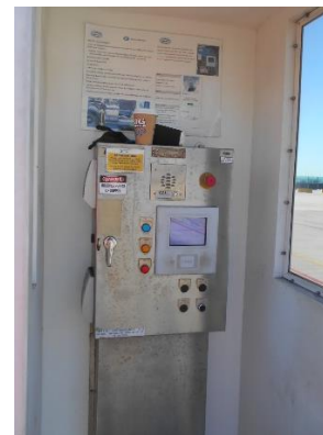
Rubbish left in the landside truck booths by the truck drivers.
