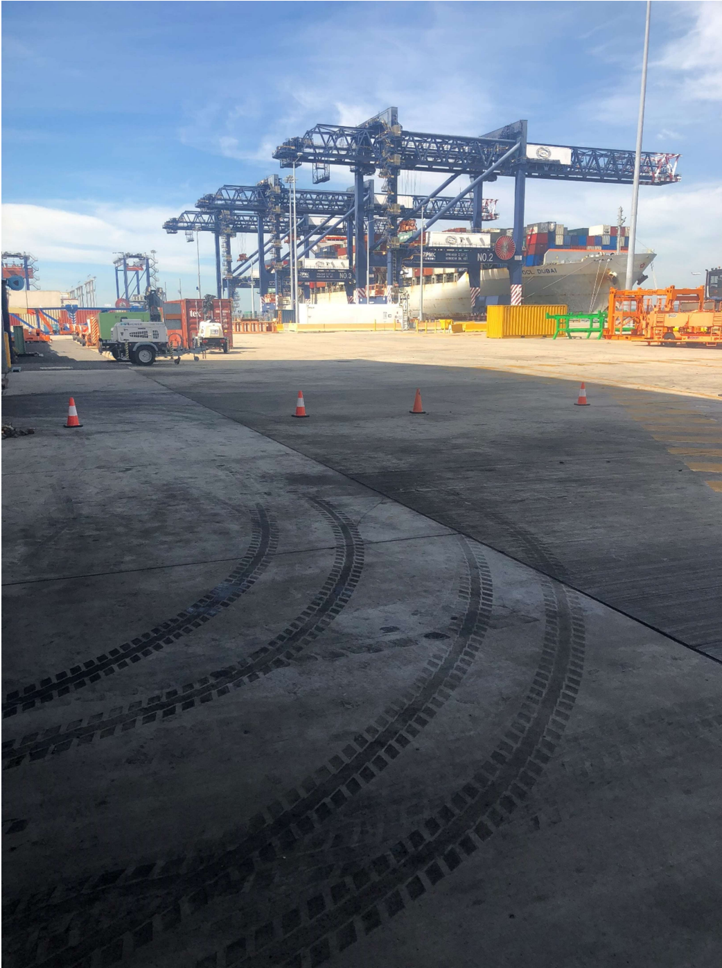
Plate 6: Wash bay area clean with no tracking of material onto concrete
