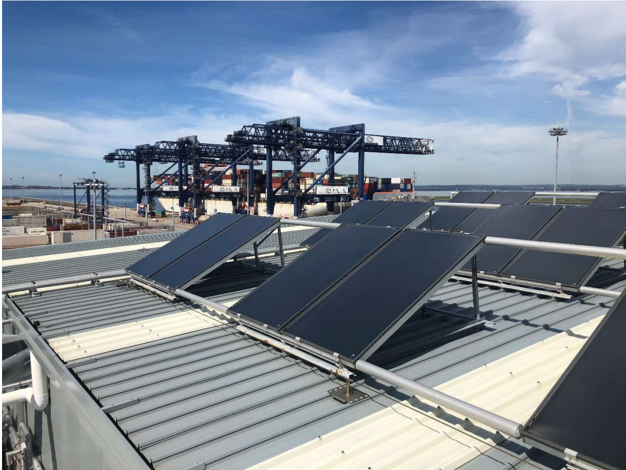
Plate 7: Solar panels on roof of workshop
