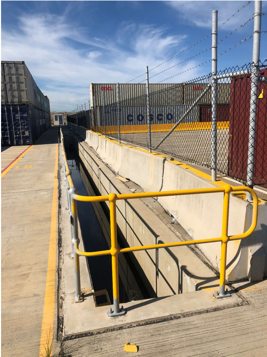
Plate 2: Collection drain behind leaking container storage area
