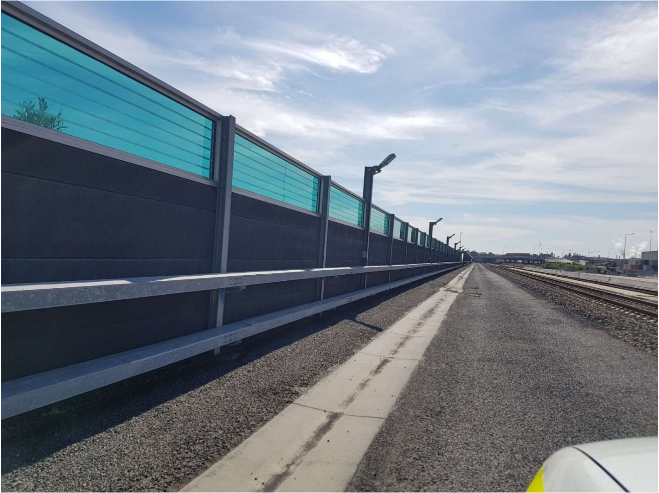
Plate 3: Noise wall close to rail tracks
