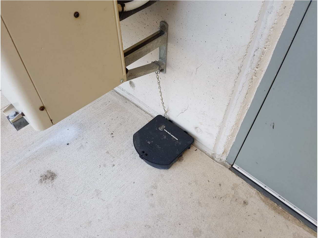
Plate 5: Pest control bait station
