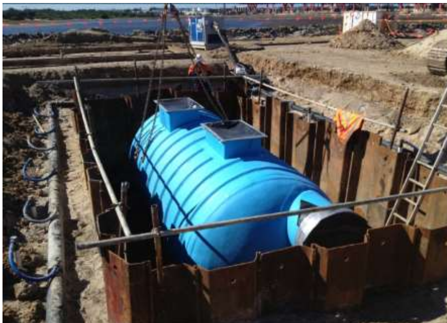
A SPEL Environmental ‘Stormceptor’ separator unit being installed during construction of the terminal in 2013.
