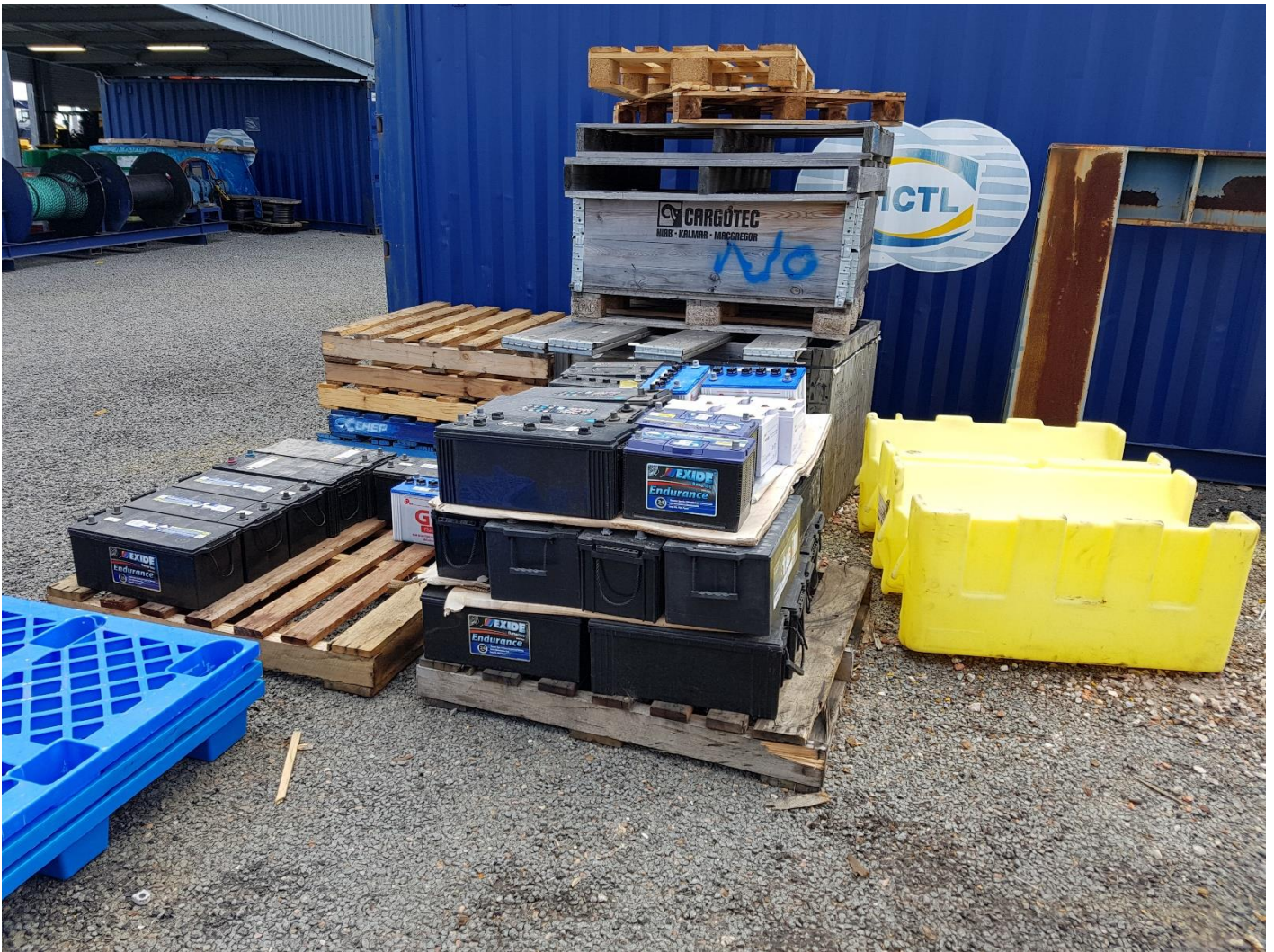
Plate 11: Batteries stored without appropriate spill containment measures
