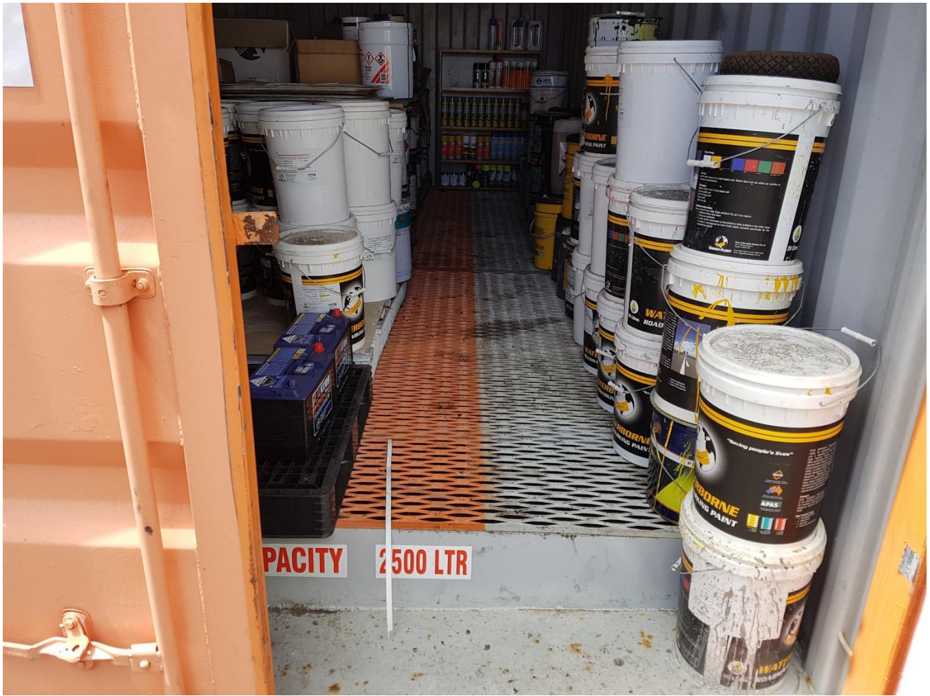
Plate 2: Paint containers, batteries & other liquids stored in bunded container
