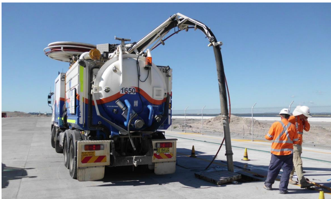
Figure 4 SQUID 7 being cleaned out by vacuum truck in December 2013 prior to handover.
