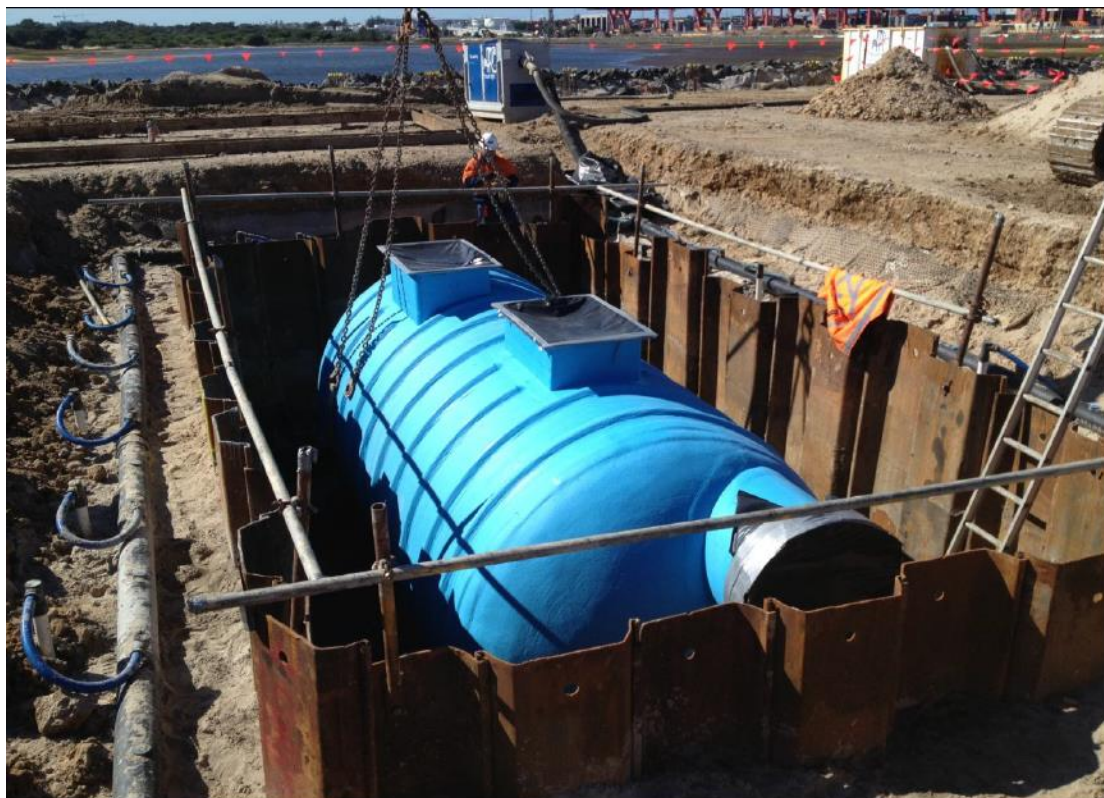
Figure 2 A SPEL Environmental ‘Stormceptor’ installed during construction of the SICTL Terminal in 2013.
