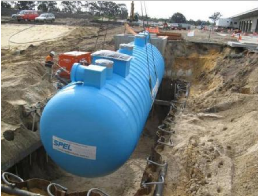
Figure 5 - SQID being installed showing cofferdam and spears
