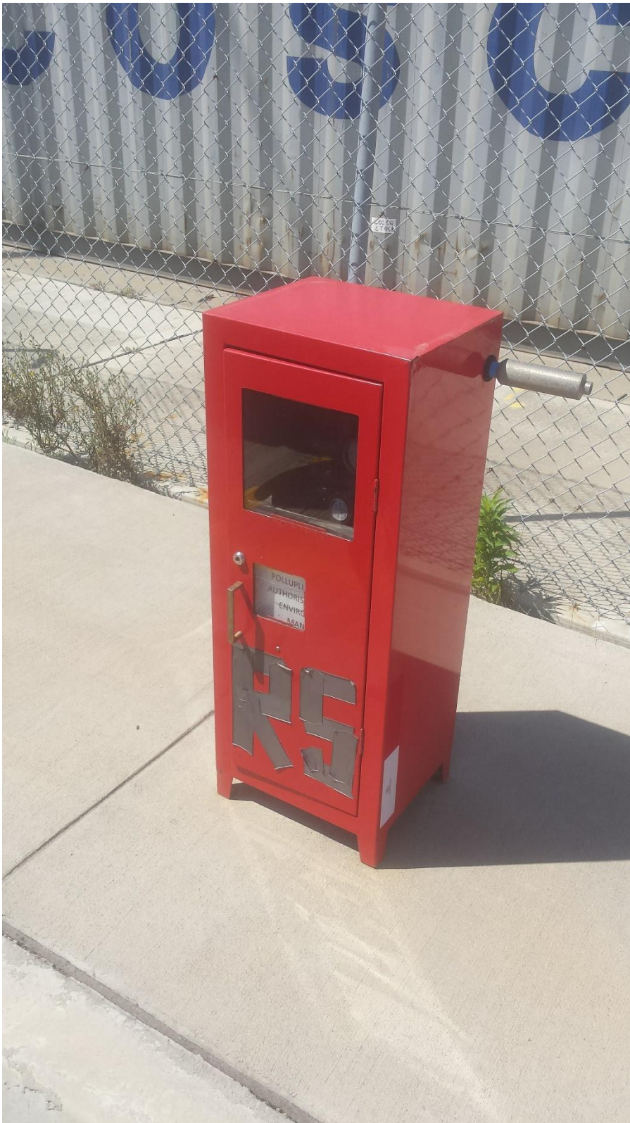
Plate 5: Polluplug stormwater pollution control device
