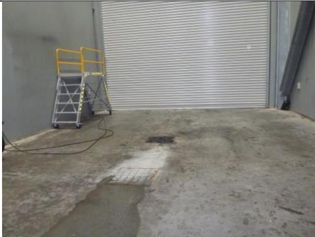
Photo 1: Plant washdown bay. Water drains to a settling tank and is treated through a coalescing plate oil water separator then discharged to sewer.
