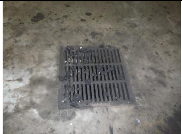
Photo 2: Close up of drain in washbay. No Sydney Water consent to discharge industrial waste water is held by the facility. Refer to EM NC 1 and IOC 1 & 2
