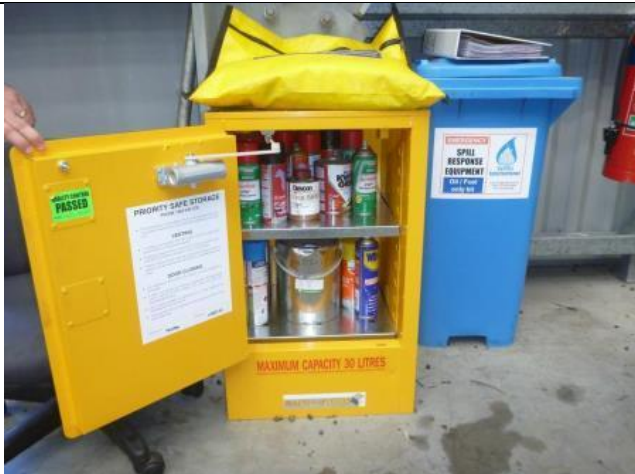
Photo 5: Storage of minor quantities of flammable substances in purpose build bunded storage cabinet ✓
