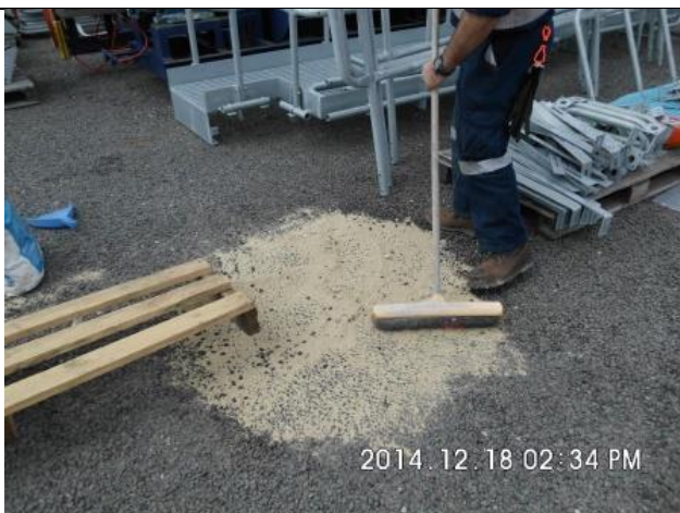
Photo 30 – clean-up of minor oil spill (refer to photo 3)
