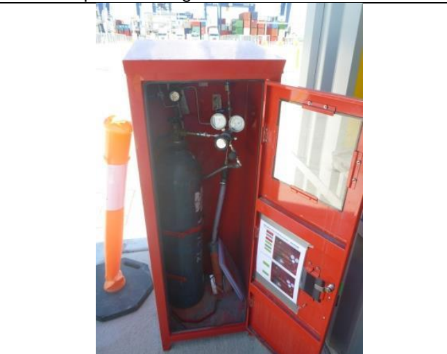
Photo 17: Pollu plug apparatus – manually operated in case of spill. Requires key to access controls ✓
