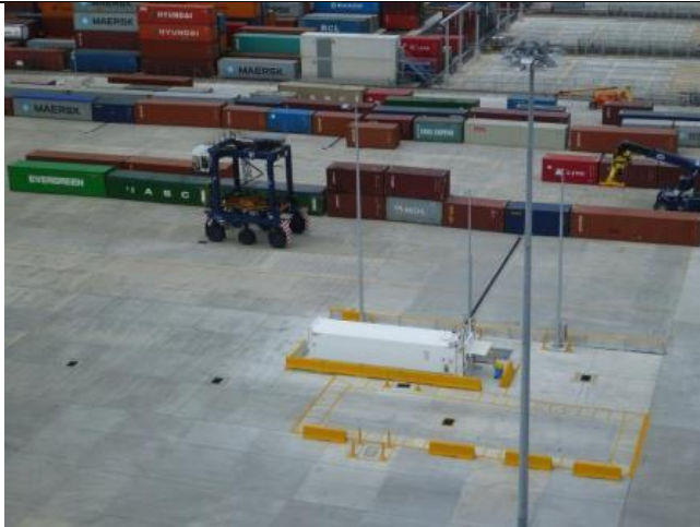
Photo 7 – View of diesel refuelling facility – area is banded, has spill kits and signage – not yet commissioned at the time of the audit. ✓
