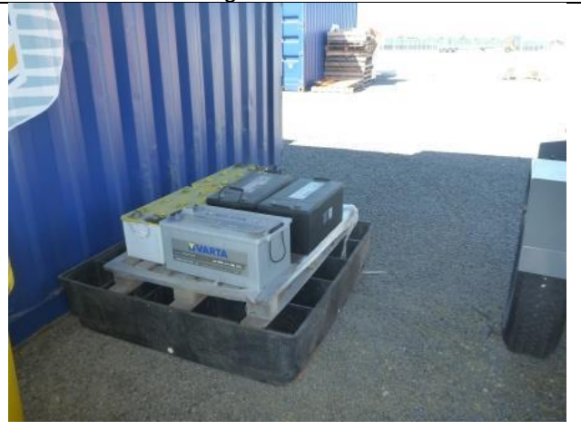
Photo 6: - Storage of batteries on bunded pallet (outside – under awning) ✓
