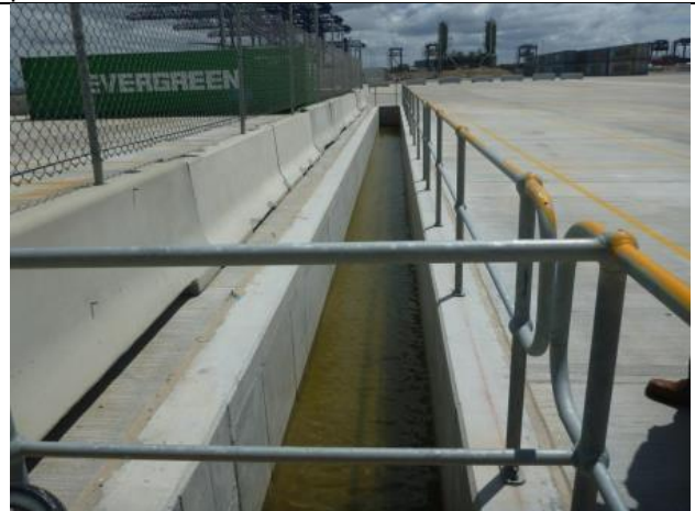
Photo 12 – Sump behind storage area for leaking containers (valve kept in closed position, clean water pumped out following rain) ✓
