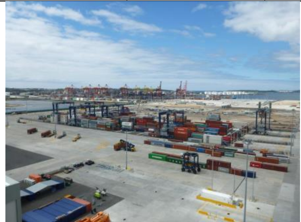
Photo 28: View of site from Quay crane. Site surface is fully sealed – minimal dust issues or roosting sites
