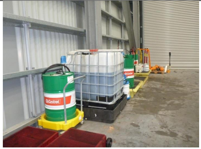
Photo 4 – Storage of oils on bunded pallets in the maintenance building ✓
