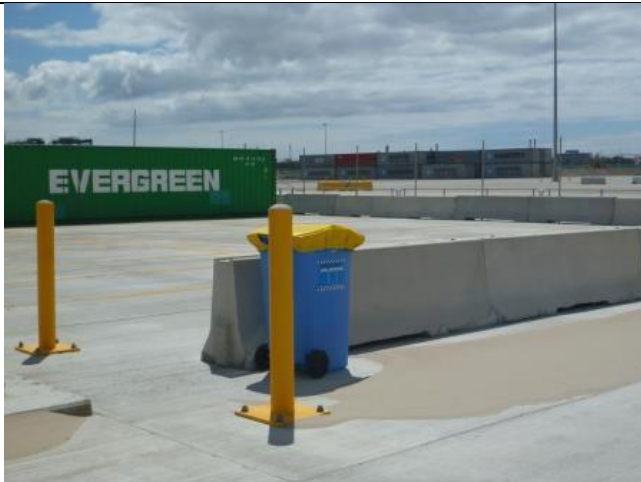
Photo 11 – Dedicated area to which leaking/potentially leaking container would be taken – drains to sump (see photo 12) ✓
