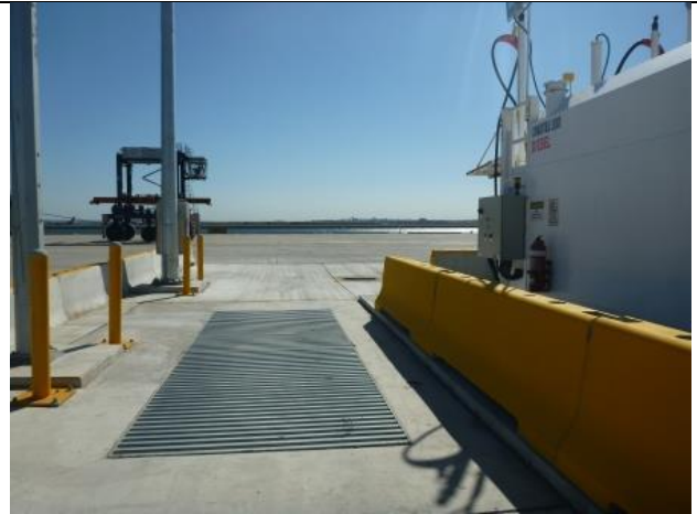
Photo 8: - Ground view of diesel refuelling facility – dedicated area for refuelling of light vehicles (plant would refuel in larger bay on other side of tank) ✓
