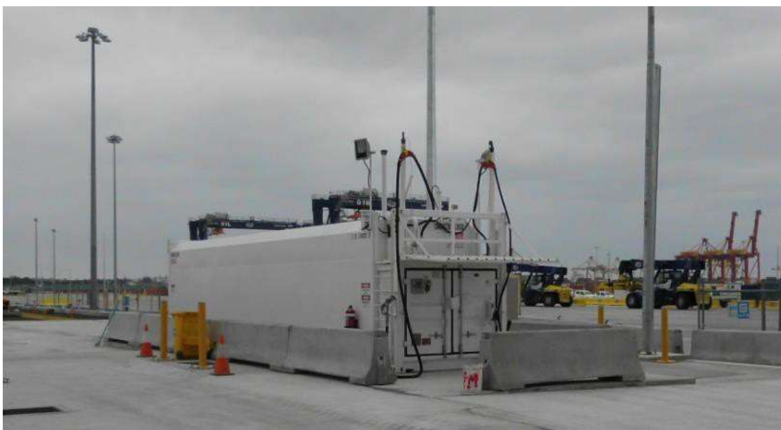
Figure 23 An example of the Transtank self-bunded diesel storage unit.
