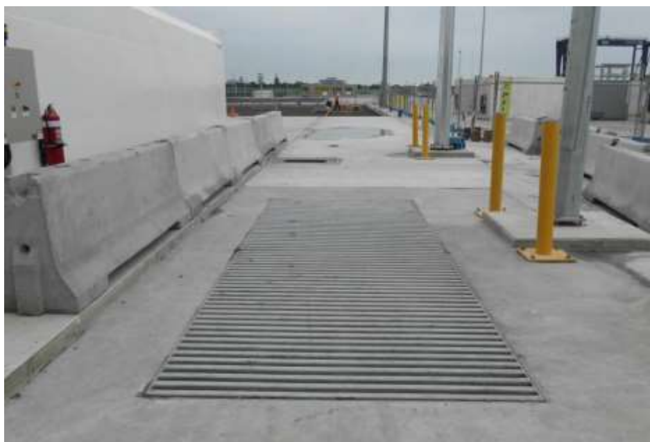
Figure 24 The tray and grate bund system for refuelling areas.
