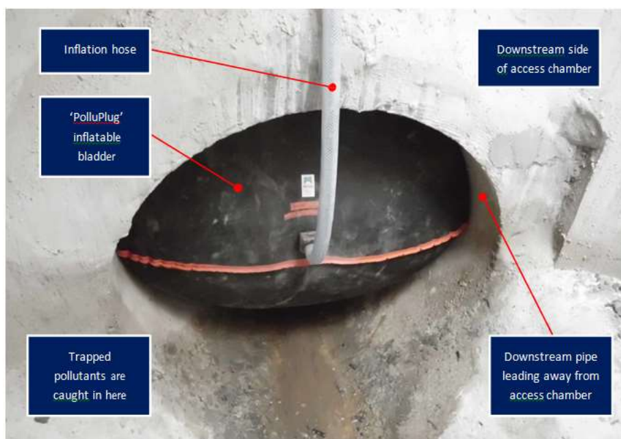
Figure 15 Looking downstream at a 'PolluPlug' inflatable bladder within the pipe draining ASC block 1. The photo was taken from within an access chamber
